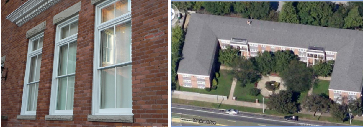
Figure 5. Philadelphia multi-family apartment building with installed low-e storm windows. Source: EERE 2013.
