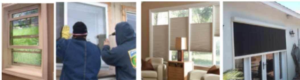
Figure 1. Window attachment retrofits (from left to right) interior operable storm window, exterior low-e storm windows, insulating cellular shades, and exterior shades. Source: PNNL, AERC.
