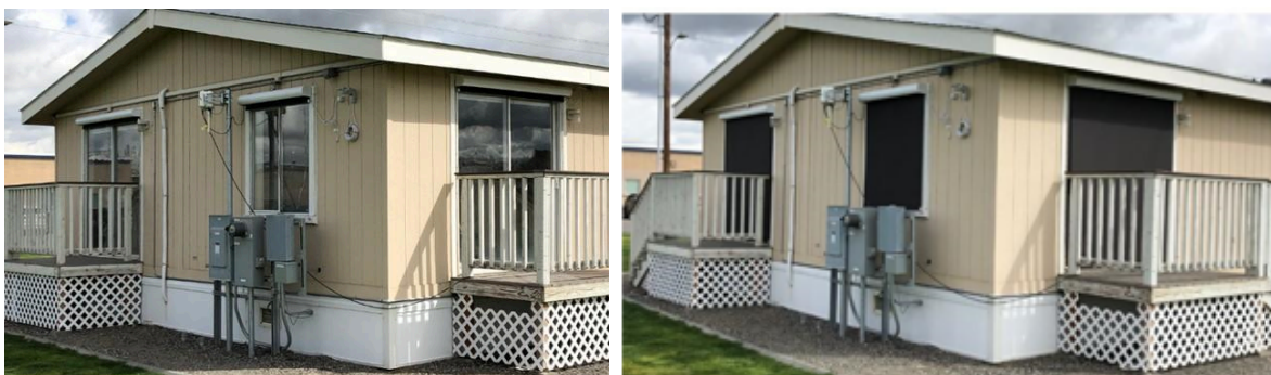
Figure 7. PNNL Lab Homes shown with exterior shades rolled up (closed) and rolled down (open). Source: Hunt and Cort 2020.
