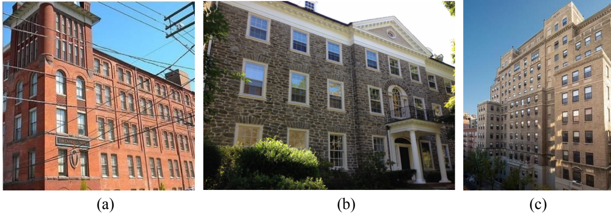
Figure 11. Examples of low-e storm windows on historic multi-family upgrades. (a) 1892 Umbrella Works, Lancaster PA - adaptive reuse to apartments, interior low-e panels. (b) Wissahickon Avenue Apartments, Chestnut Hill, PA - exterior low-e storm windows. (c) 1929 French Apartments, New York City, NY - interior operable low-e panels. Photos courtesy of QuantaPanel.
